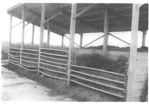
Figure 5. This simple four-bin swine mortality composting unity includes space for dry storage of cover material behind the bins. (Photo by Palmer Holden, Iowa State University.)
